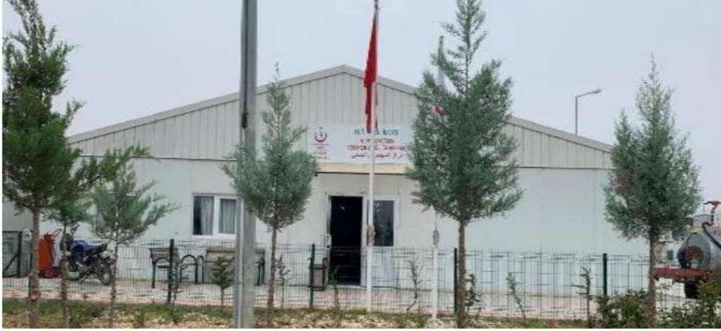
Figure 3. 1. Boynuyöğün Temporary Accommodation Centre Health Facility. 123
